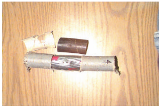
Textile-Covered RHW Cable With Strand Displacement Typical of B-Strand Failure Mechanism
