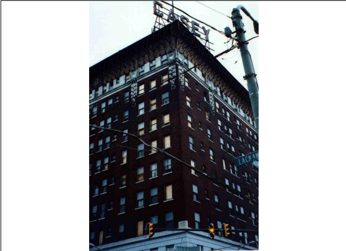
Figure 3 The Casey Hotel before demolition
