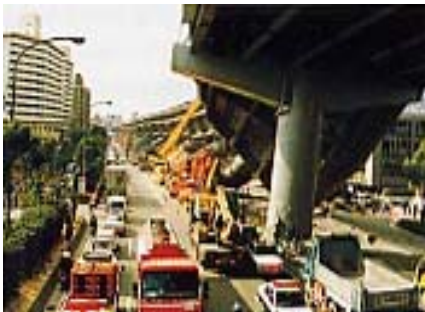
Figure 21 Damage to battery stand legs in San Francisco is similar to the damage experienced in the columns of the collapsed sections of the Hanshin Expressway during the 1995 earthquake in Kobe, Japan.
