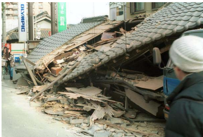
Figure 4 failed homes during the 1995 Hyogoken-Nanbu earthquake in Kobe Japan caused by the top-heavy nature of their construction that could not withstand soil displacement taking the structure out of plumb.
