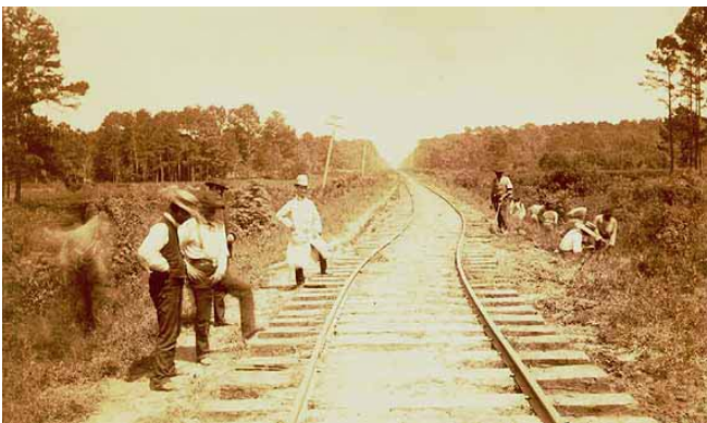
Figure 7 Railroad track displacement from an earthquake in Charlotte, NC. The track was straight before the event.
